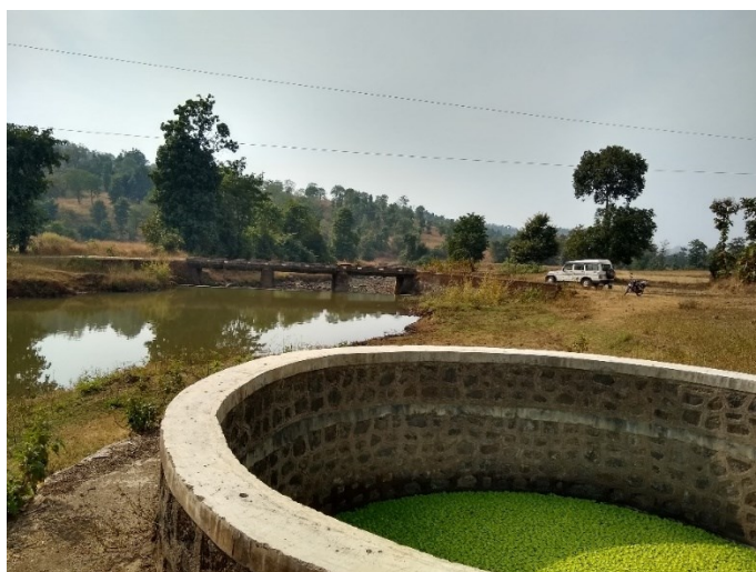
Figure 29: Condition of well 1 containing hyacinth growth
